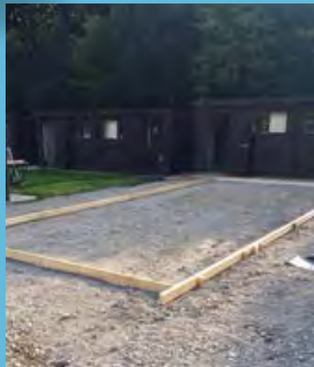
New kennels at the back and foundations for a new block.
