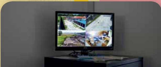
A new state-of-the-art CCTV system was installed.
