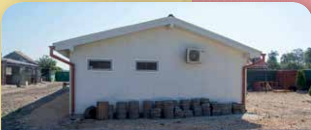
The New veterinary centre being finished off.
