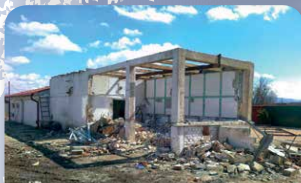
Work has started to renovate the vet surgery at the Victory shelter in Brasov.
